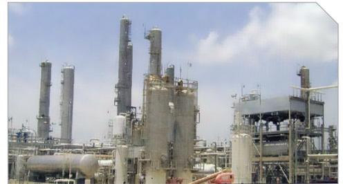
The Mont Belvieu plant operates 25 York centrifugal compressors in the 4000 hp (2982 kW) class, 15 of which are in DIB Isobutane service. It also operates over 500 pumps ranging from 10 to 600 hp (7.45 to 447 kW), 90% of which run at 3600 rpm.
