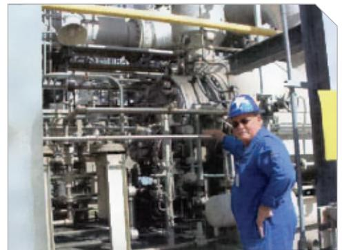
Maintenance Foreman David Wright checked out this two-stage York centrifugal compressor model M255B on Isobutane service coupled up to a Solar T4702S Centaur gas turbine.
